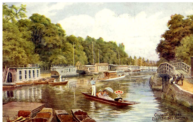
'College Barges, Folly Bridge, Oxford', by A. R. Quinton, 1914.
